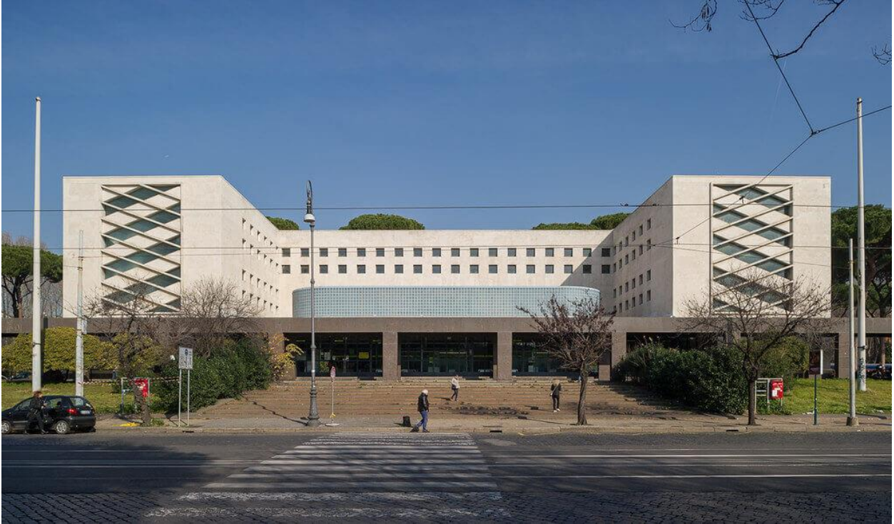
Figure 14 Facade of the Ufficio Postale in via Marmorata 4, Rome
